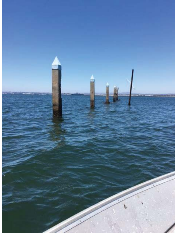
Photo 3: Northerly Tire Island Piles.
