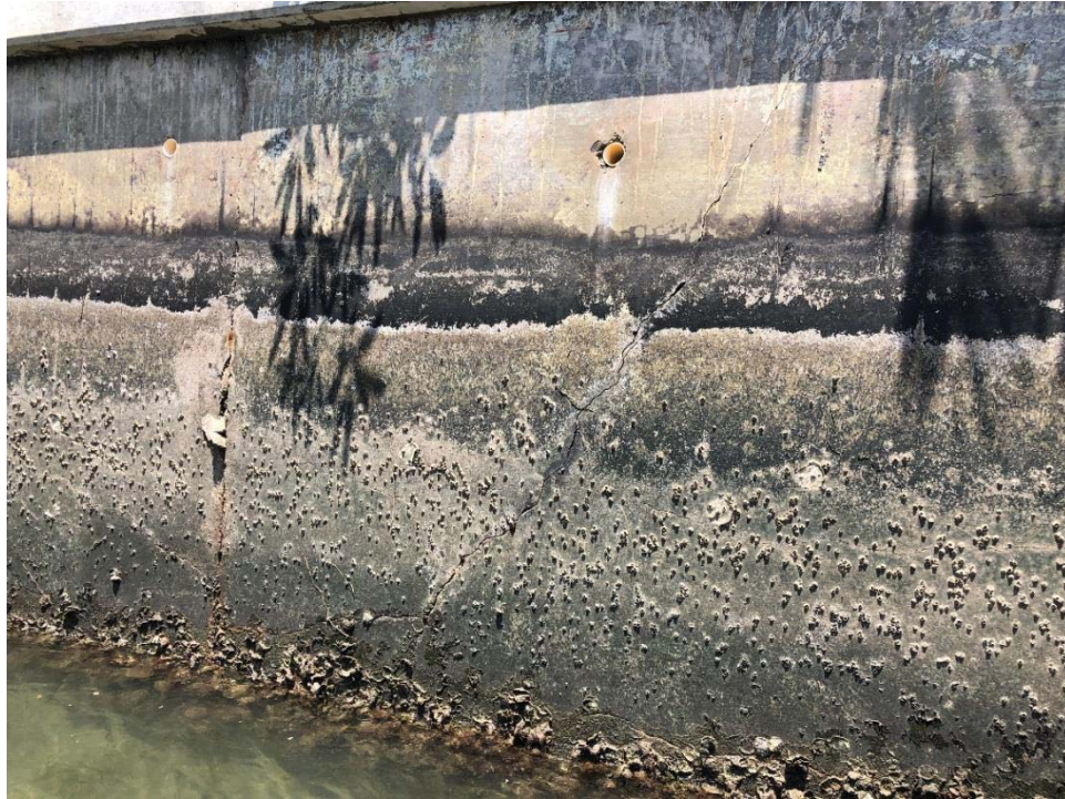
Photo 1: Spinnaker Way, Lot 5. Cracks in eastern panel.
