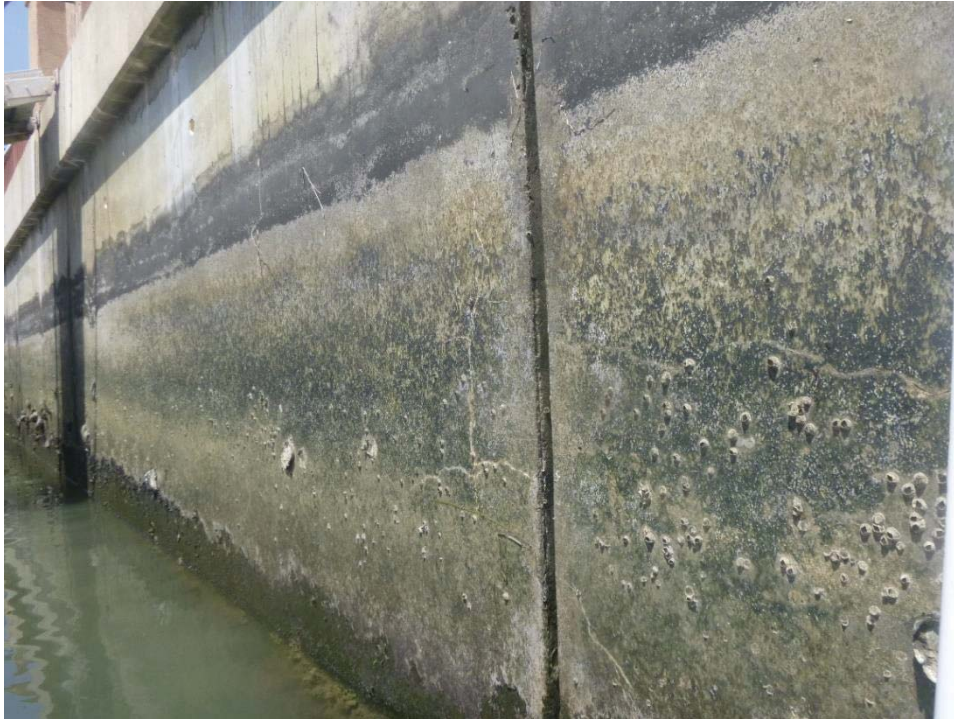
Photo 3: Blue Anchor Cay, Lot 28, Panel 2. Separation between panels.
