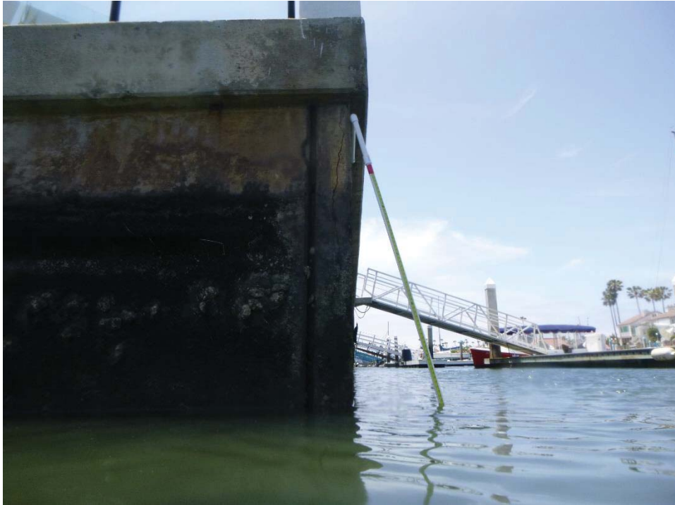
Photo 7: Blue Anchor Cay, large vertical crack along the northerly panel angle point on Lot 17. Northwesternly panel separating from adjacent easterly panel.
