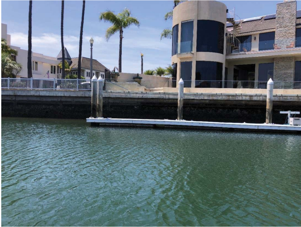
Photo 9: Spinnaker Way, north side of Lot 4. Steel whaler on north side.
