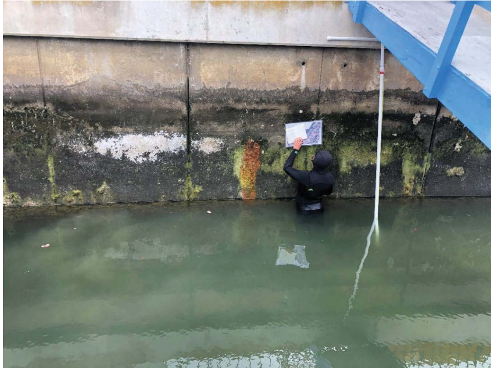
Photo 3: Catspaw Cape, west of Lot 55, public gangway. Rust stains east and west of gangway.
