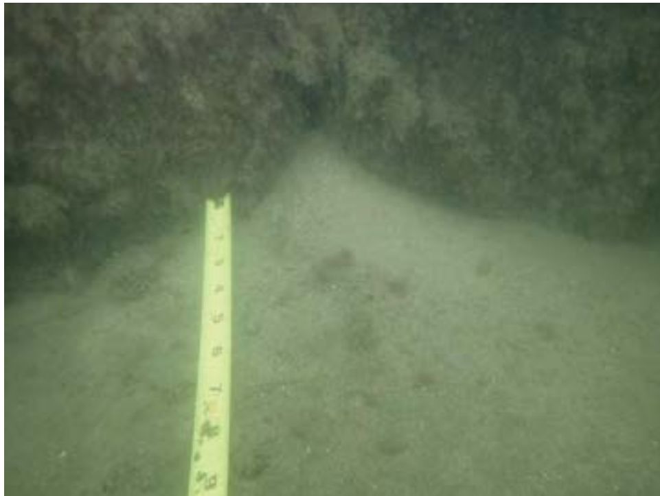
Photo 8: Antigua Court, 20 feet east of northwest corner. 6-inch-high talus pile.
