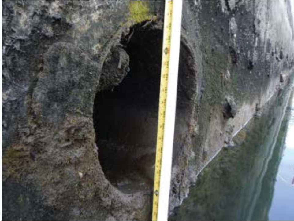
Photo 15: Antigua Court, South Side, Lot 19/21. 14-inch storm drain under gangway at P/L.
