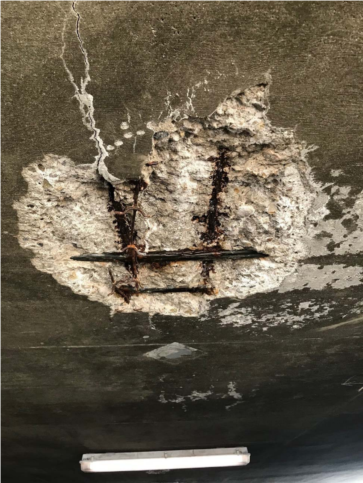
2022 0124 Photo 006 Garage Overhead SE Corner
